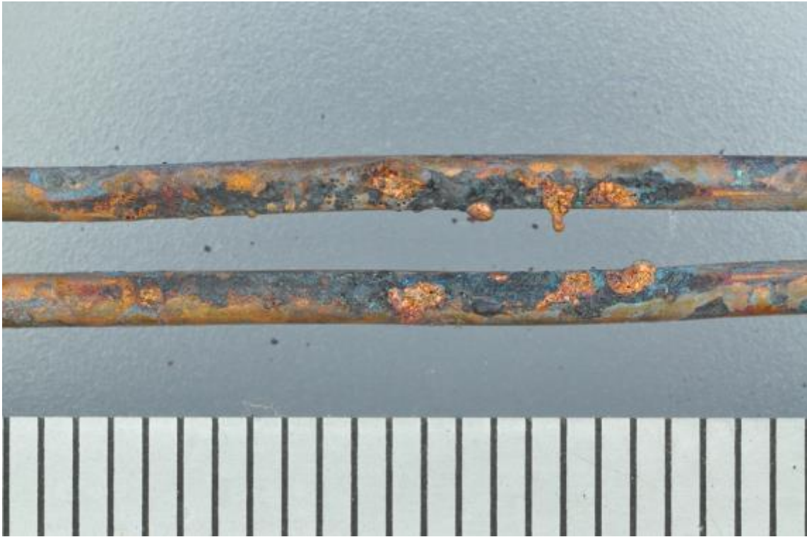
Figure 4.9.(b) Arc marks after conductor has been separated.
