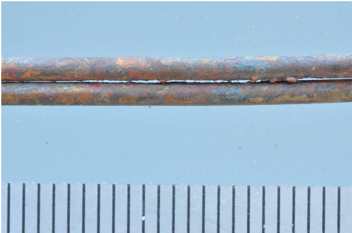
Figure 4.12.(a) Arc marks on VVF2 conductor.
